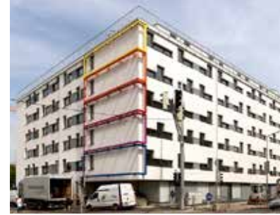
Photos Building progress WGA ZT GmbH
