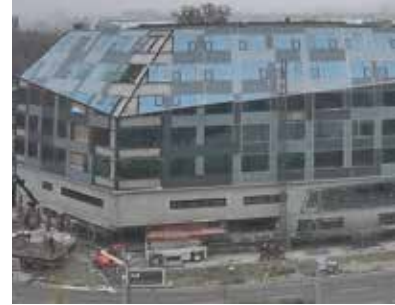
Photos Building progress: WGA ZT GmbH
