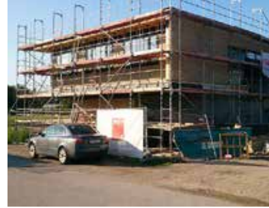
Photos Building progress WGA ZT GmbH
