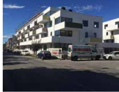
Photos Building progress: WGA ZT GmbH
