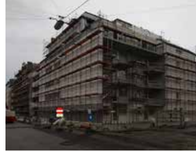
Photos Building progress: WGA ZT GmbH
