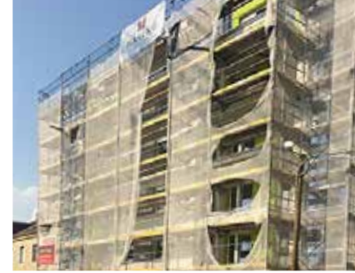
Photos Building progress: WGA ZT GmbH
