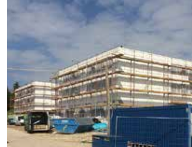
Photos Building progress: WGA ZT GmbH
