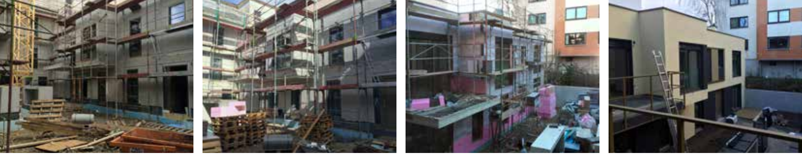
Photos construction progress: WGA ZT GmbH
