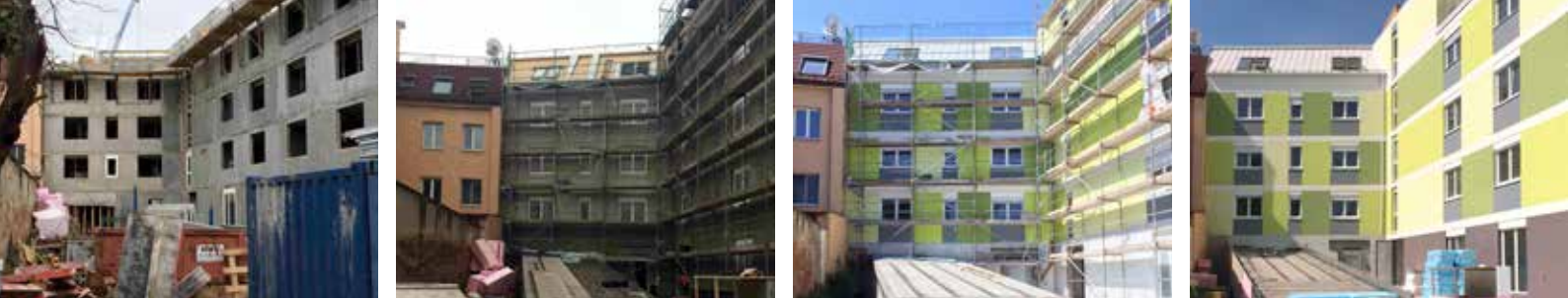
Photos construction progress: WGA ZT GmbH
