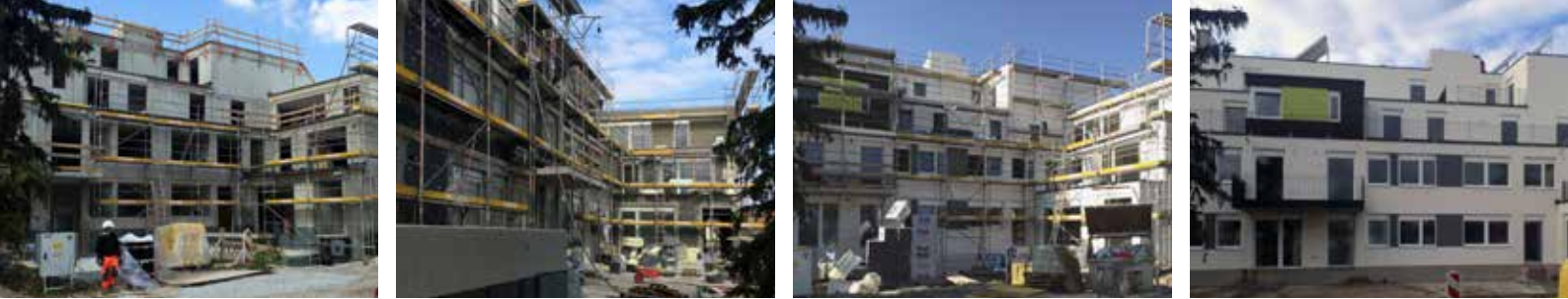
Photos construction progress: WGA ZT GmbH
