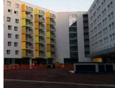
Photos construction progress: WGA ZT GmbH
