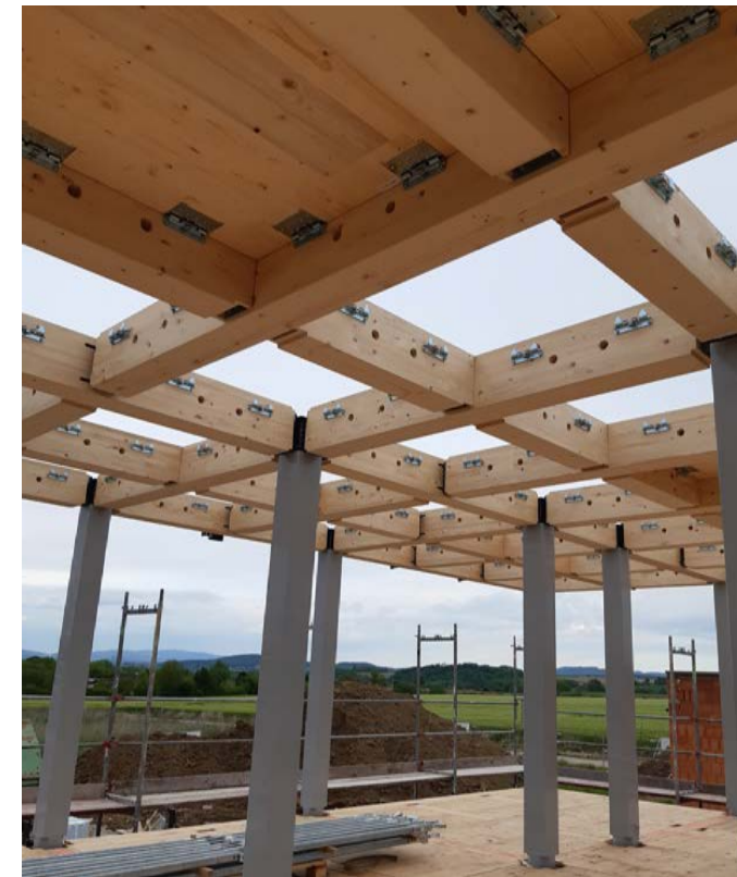
© Lukas Lang Building Technologies GmbH
