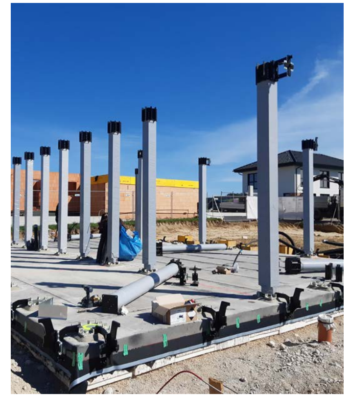
© Lukas Lang Building Technologies GmbH
